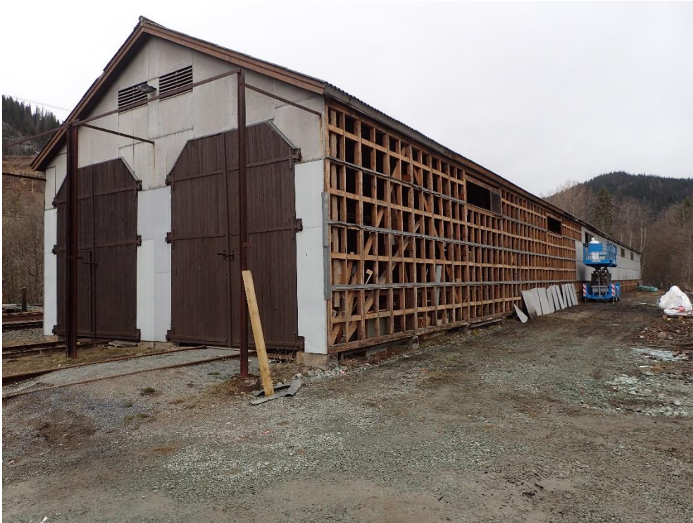
24 april 2020. Natostallen under demontering.
